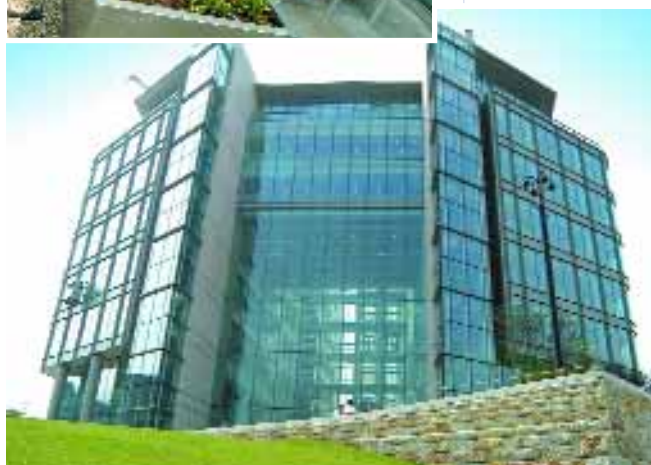
Above left: sixth floor planters Left: retaining wall with limestone rockface cladding
